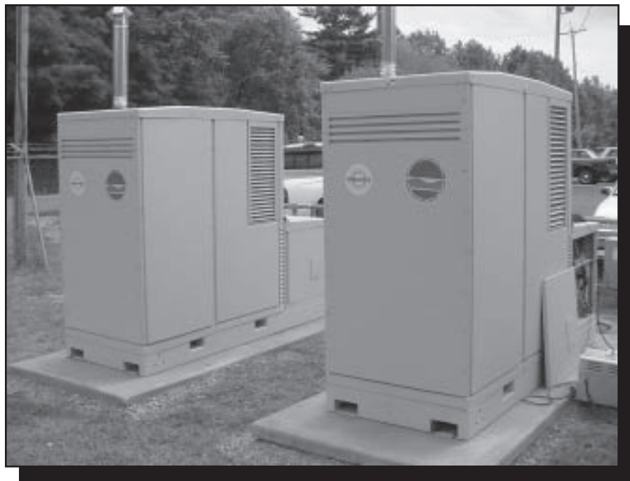
Figure 1—Moderate-size fuel cells can provide continuous or emergency power for homes or businesses.
