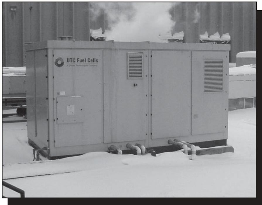
Figure 4—Steam vents from the top of a 200-kilowatt, model PC 25 fuel cell manufactured by UTC Fuel Cells. The unit can produce uninterruptible power for critical needs such as hospital life support equipment, computer centers, or emergency services, in addition to providing electrical power for more ordinary uses. —Photo courtesy of Concurrent Technologies Corp., Johnstown, PA.
