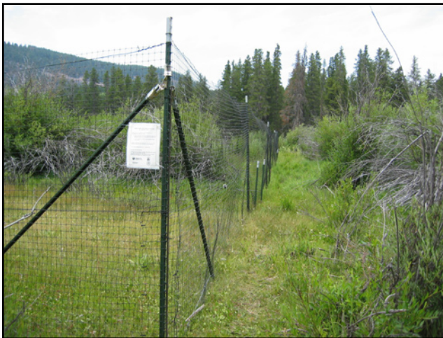
Figure 1—This moose enclosure near the Middle Fork of Rock Creek in Montana uses 10-foot-long metal T-posts driven 2½ feet deep to support polypropylene mesh fencing.
