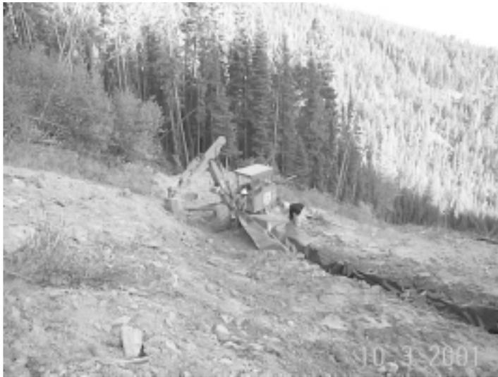
**Figure 5.** *Installing HDPE liner over bermed ditch to divert surface water runoff from the landslide.*
