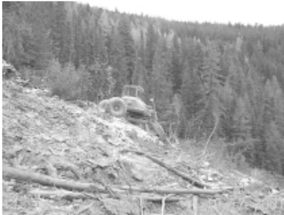
**Figure 8.** Spider hoe excavator in depositional zone, located between the upper and lower roads.
