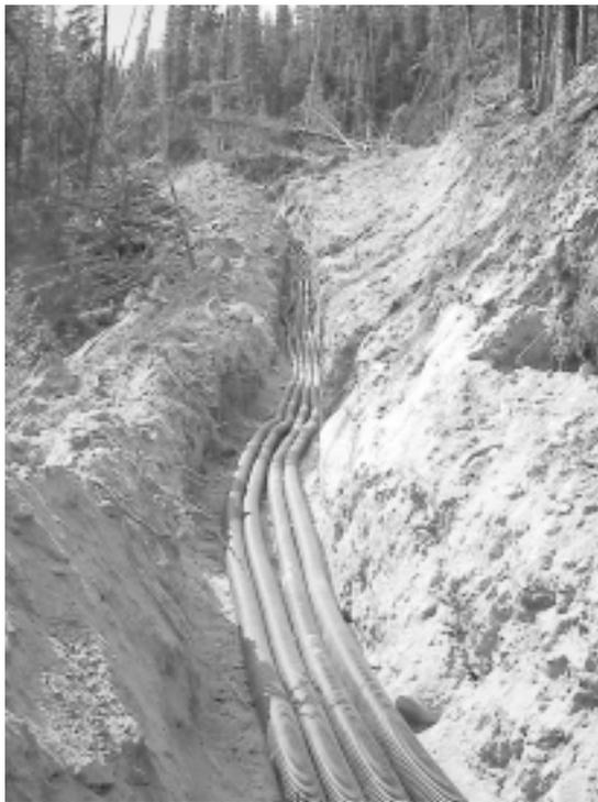
**Figure 4.** *Collector pipes that drain upper site, located along west pressure ridge.*
