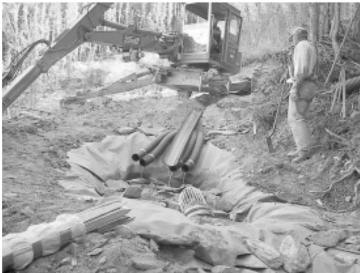
**Figure 6.** *Monitoring station to measure ground water and surface water flows drained from the middle site.*
