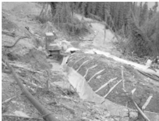
**Figure 7.** Excavation for Eljen drain located directly below headscarp. Note trench cave-in onto Eljen drain, mid-photo.
