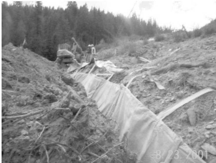
**Figure 2.** Installation of Eljen drains in depositional zone.
