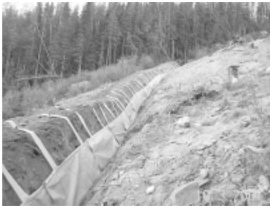
**Figure 3.** *Eljen drain panels staked at grade, middle site.*
