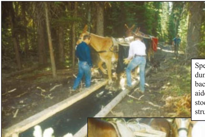
Special panniers make it easier to carry and dump gravel during trail construction in the backcountry. Trail construction is also aided by drawings of equipment for pack stock, a series of videos, and a trail construction notebook published by the center.
