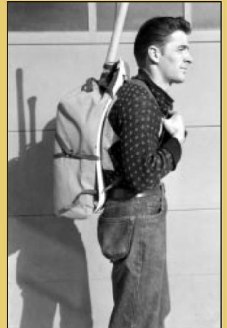
Contoured fiberglass pack boards replaced wooden models, making the task of carrying fire packs a little easier.
