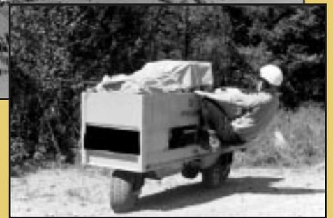
*Gyroscopes kept this prototype cargo carrier upright, even when someone tried to pull it over. The goal was to find a way to transport ore from backcountry mines on trails rather than roads. The electronic controllers available during the 1960s did not respond quickly enough when the carrier hit large rocks. Once the carrier was part of the way over, the gyroscope threw it to the ground. The project was abandoned. With modern electronics, these carriers would be more likely to succeed.*
