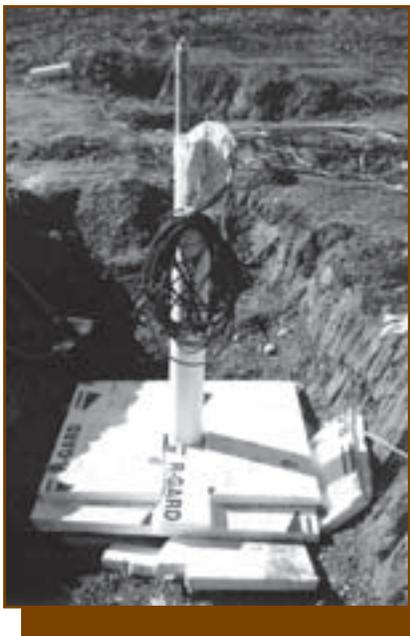
Figure 15—Insulation installed around a typical SVE extraction well.
