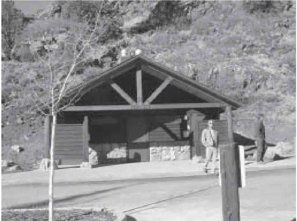
Figure 1. Fish Creek Falls Recreation Vault Evaporator Toilet Building (front view)
