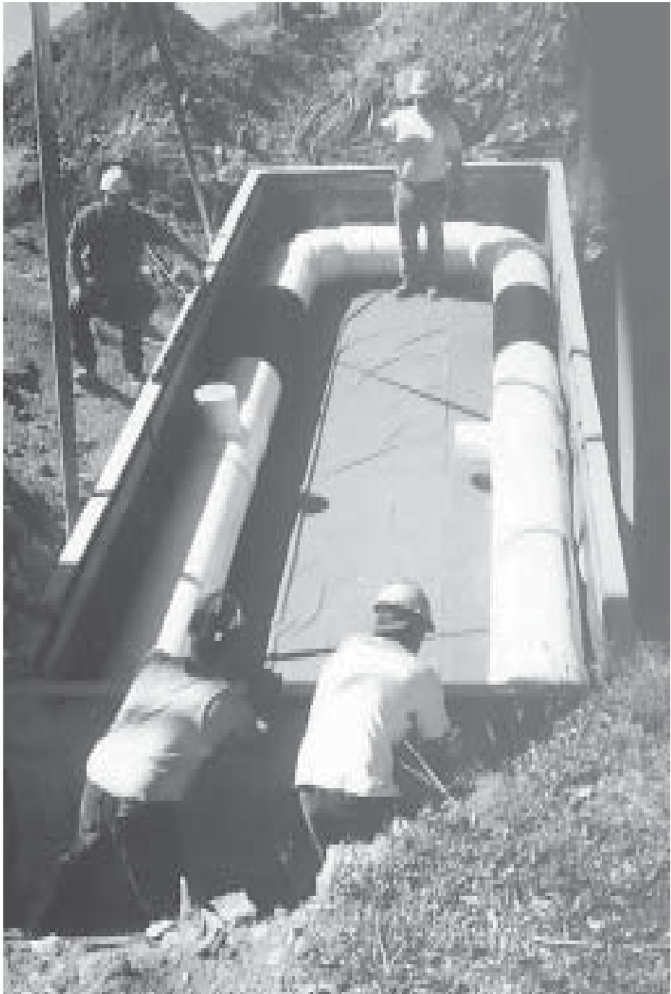
Figure 3. Installation of the vault evaporator. Liquid enters the perimeter pipe and fans force air through the pipe to promote evaporation.
