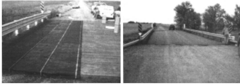
**Figure 10 (left).** Bridge deck with moisture barrier being placed.
