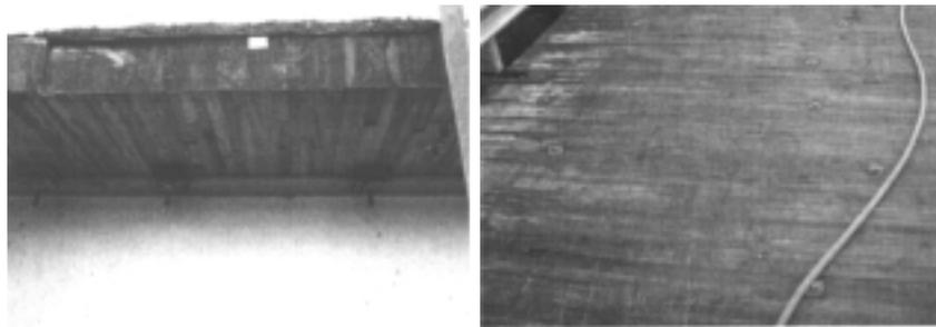
**Figure 8 (left).** End view of deck panel attached to steel girder with clips.
