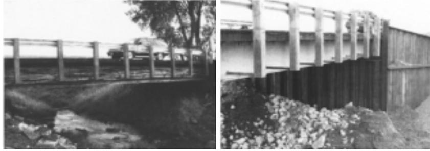
**Figure 6 (left).** Panel deck with wood beam design.
