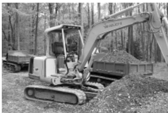
Figure 3. A mini excavator in action.
