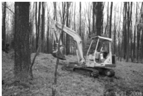
Figure 1. Using mini excavators proved to be quick and efficient.
