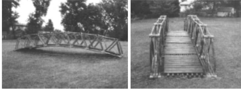
**Figure 12 (left).** Side view of LPSA bridge with 35 foot span.
