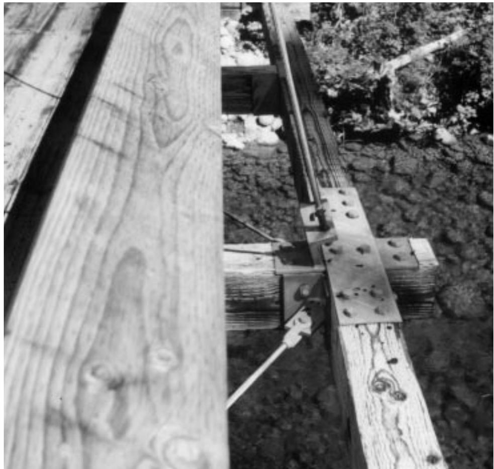
**Figure 3.** Typical connection of the deck system and suspension cables.
