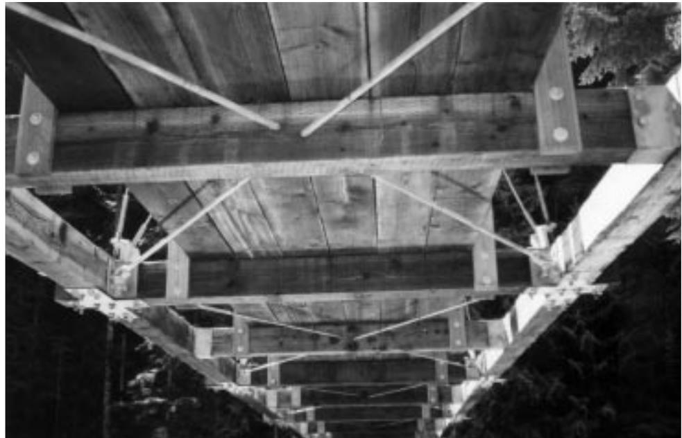
**Figure 5.** A view of the deck frame from below, showing cross bracing with rods.
