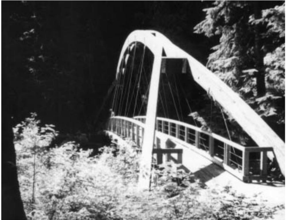
**Figure 2.** View of the arch showing the taper from the wide base to the narrow center spline.
