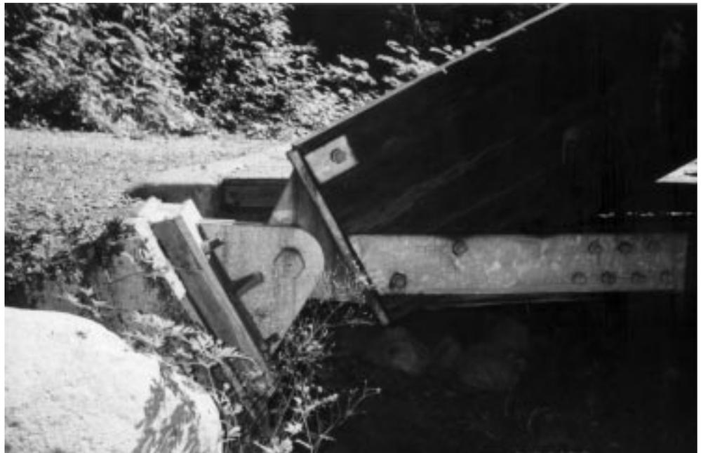
**Figure 4.** Footing pedestal and anchored hinge connection.
