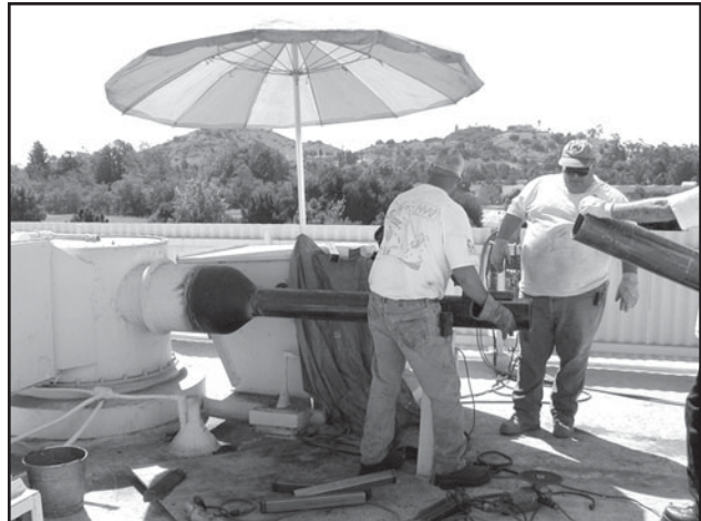
Construction during the upgrade of the spark arrester laboratory at SDTDC.
