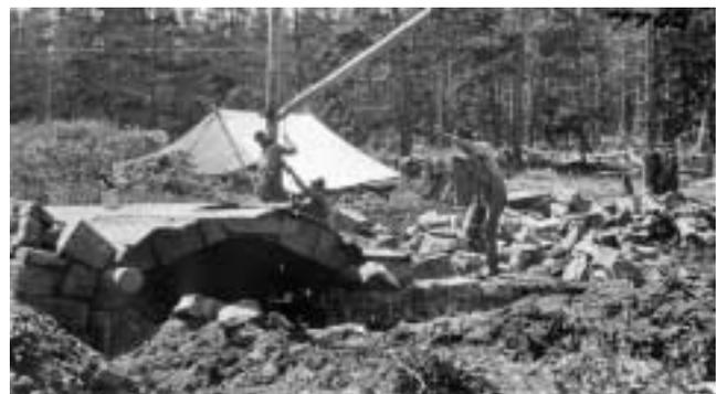
Figure 14—Neihart Masonry Arch circa 1916. Note the “ginpole” for moving heavy stones into place.
