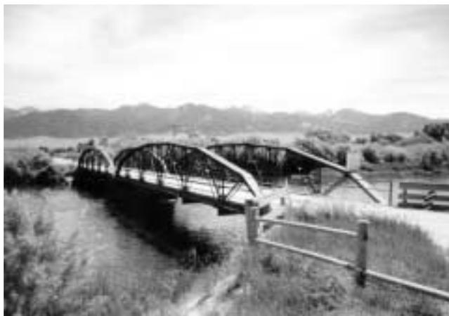
Figure 21—Jefferson River Bridge at Silver Star, MT. This riveted Warren pony-truss bridge has been “adopted” by the Bonner Development Group and will soon be relocated to a site crossing an overflow channel of the Clark Fork River near Bonner, MT.
