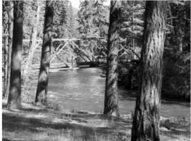
Figure 8—Minam River Horse Trail Bridge on the Wallowa-Whitman National Forest. This Howe through-truss bridge was completed in 1945.
