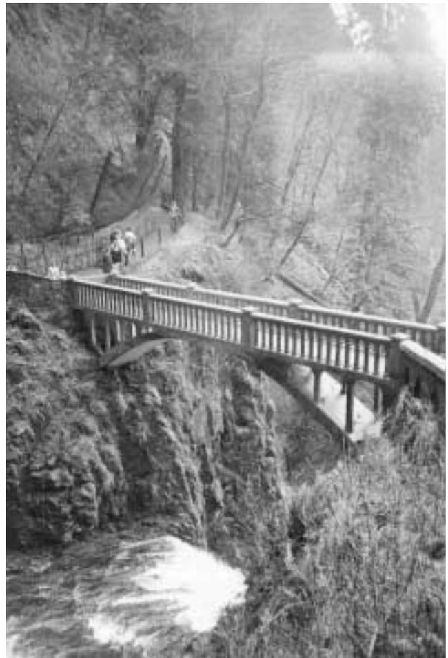
Figures 9, 10—Multnomah Falls Trail Bridge (Benson Footbridge) on the Mount Hood National Forest in Oregon. This open-spandrel concrete arch bridge was constructed in 1914.
