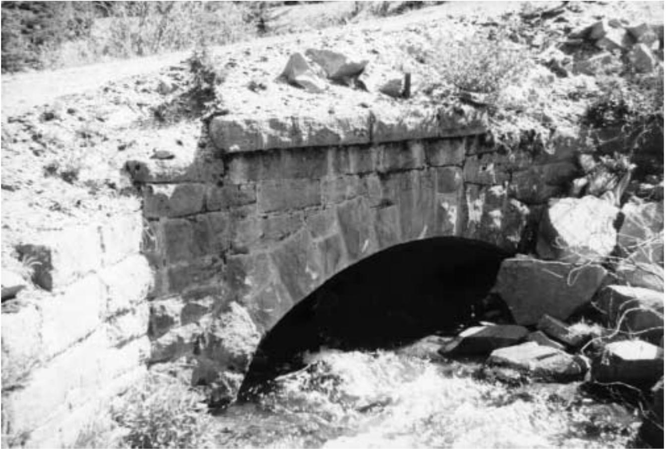
*Figure 16—Neihart Masonry Arch circa 1999. This arch is not currently listed on the National Register of Historic Places and is not used as a road or trail bridge.*
