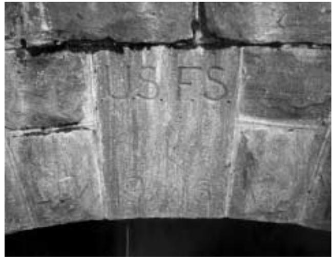
Figure 13—Neihart Masonry Arch Bridge. The Neihart Arch on the Lewis and Clark National Forest in Montana was constructed in 1916. Note the USDA Forest Service shield and date cut into the keystone.
