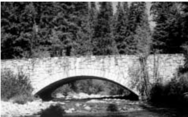
Figure 7—Deep Creek Arch Bridge on the Bitterroot National Forest in Idaho. The Civilian Conservation Corps constructed this masonry arch in the late 1930's under the direction of Art Kahl. Photo by Dan Summerfield.
