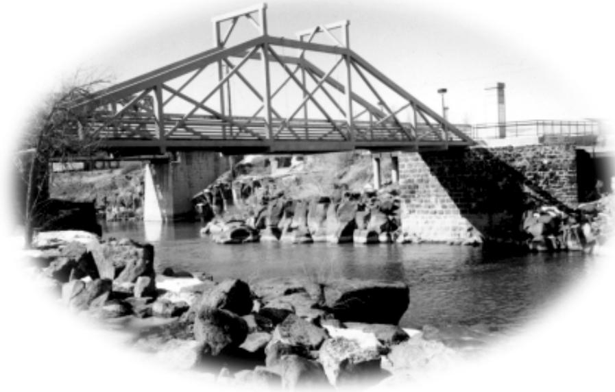
*This bridge is a steel replica of the 83-foot log toll bridge Matt Taylor built across the Snake River during 1865. Freighters and miners crossed the log bridge on their way from Salt Lake City to the gold fields in the north, passing through what is now Idaho Falls, ID. The bridge, built in 1997, is not eligible for listing on the National Register of Historic Places.*
