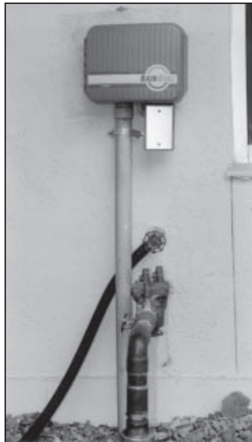
Figure 6—A timer for controlling irrigation sprinklers. If water is supplied by a well or electric pump, irrigating early in the morning or at night instead of during the middle of the day will lower peak electrical demand, reducing the electric bill.
