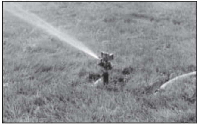
Figure 5—Sprinklers supplied by a well or pump using an electric motor increase electrical demand charges when they are used during the day.
