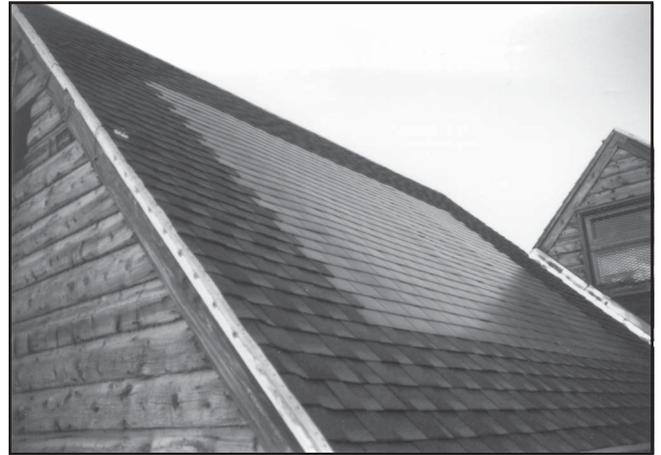
Figure 9—Photovoltaic cells on the roof of a Forest Service building. Photovoltaic cells produce power during the daytime when the peak demand for electricity usually occurs.
