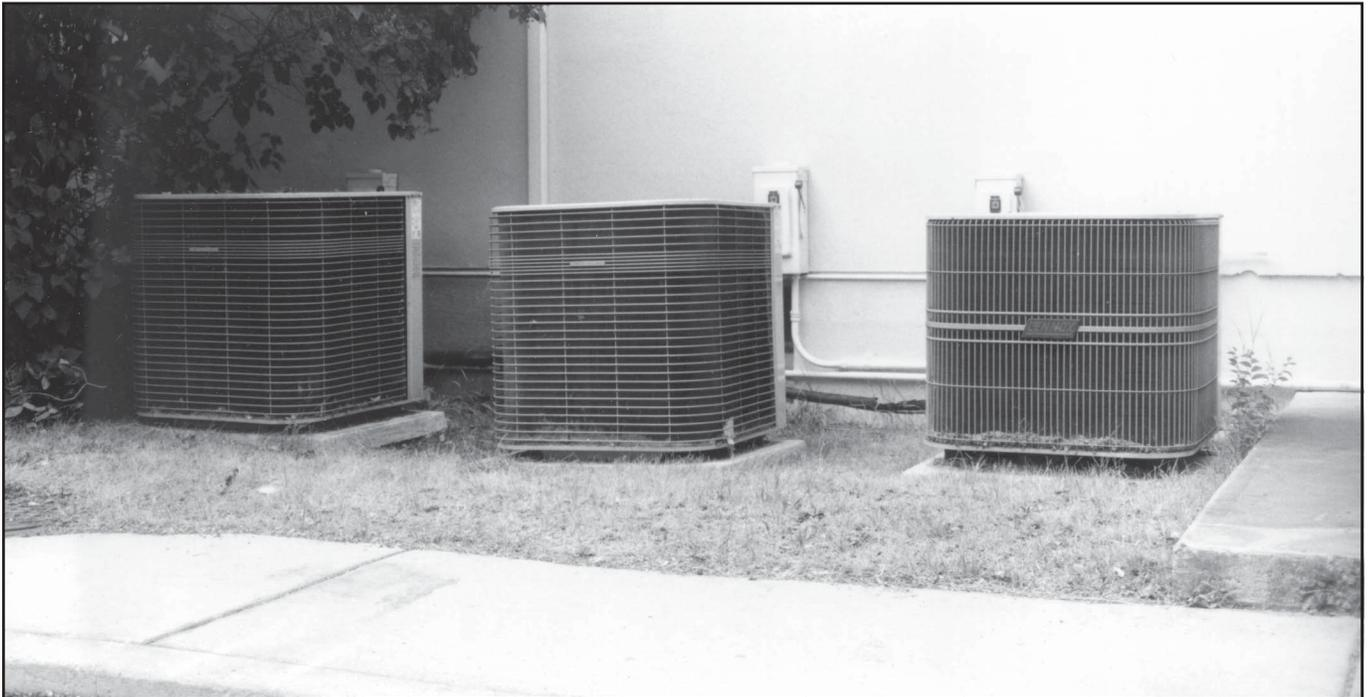
Figure 7—Three of MTDC's six air-conditioning compressors. Installing a controller that would prevent all the compressors from operating at the same time would lower MTDC's peak electrical demand.
