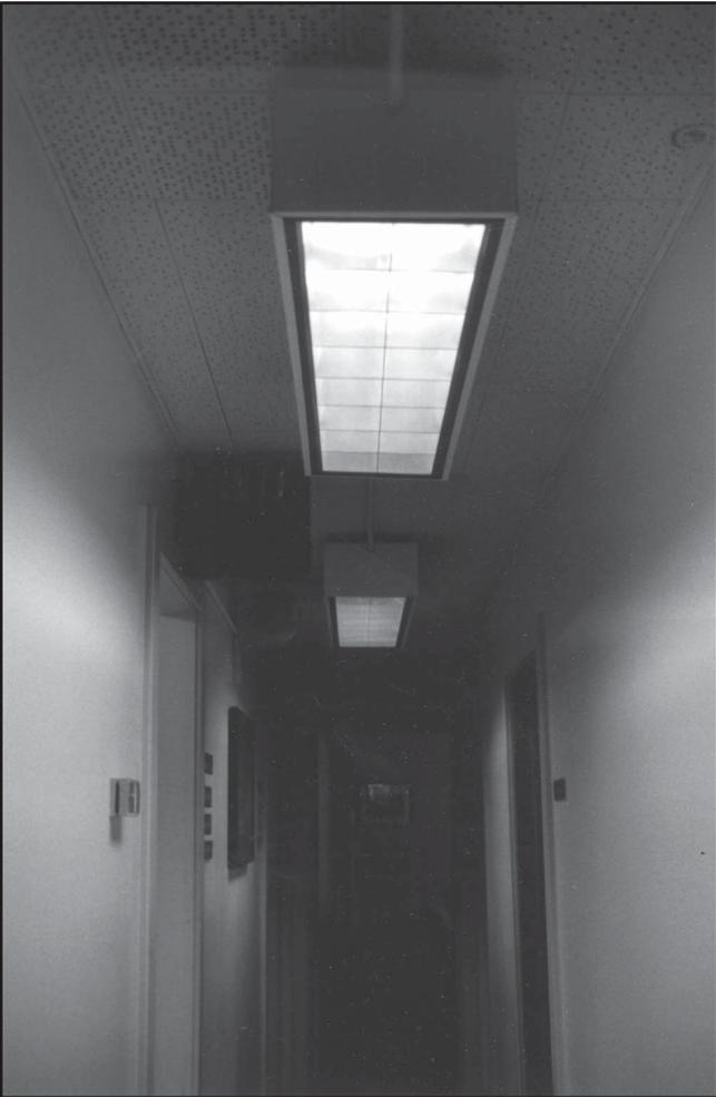
Figure 4—Light fixtures with energy-efficient T8 fluorescent lamps and electronic ballasts save energy and reduce peak demand.
