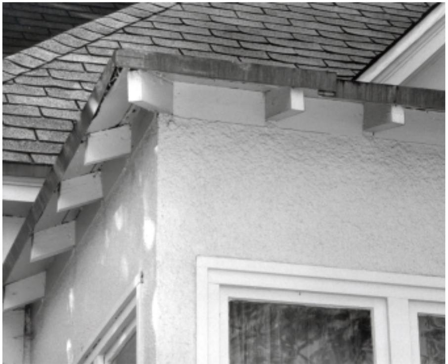
Figure 4—Stucco siding provides effective protection against the elements.
