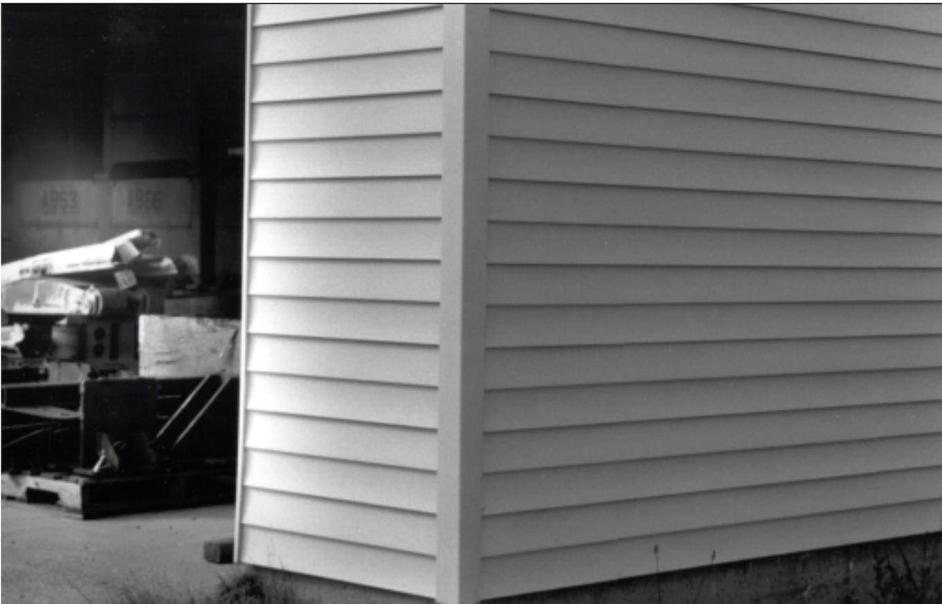
Figure 5—Vinyl siding comes in a variety of textures, colors, and sizes.
