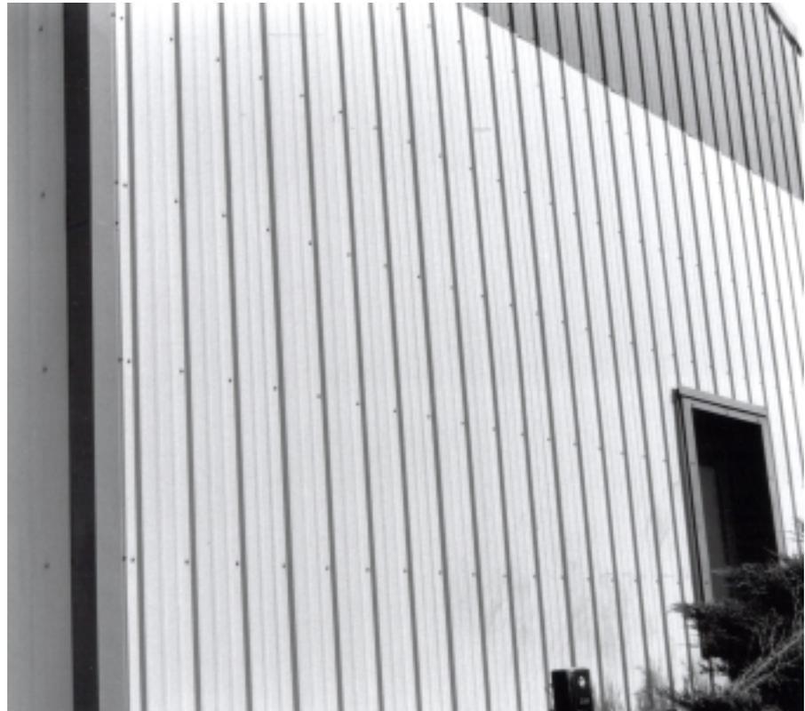
Figure 2—MTDC’s garage uses vertically arranged steel siding.
