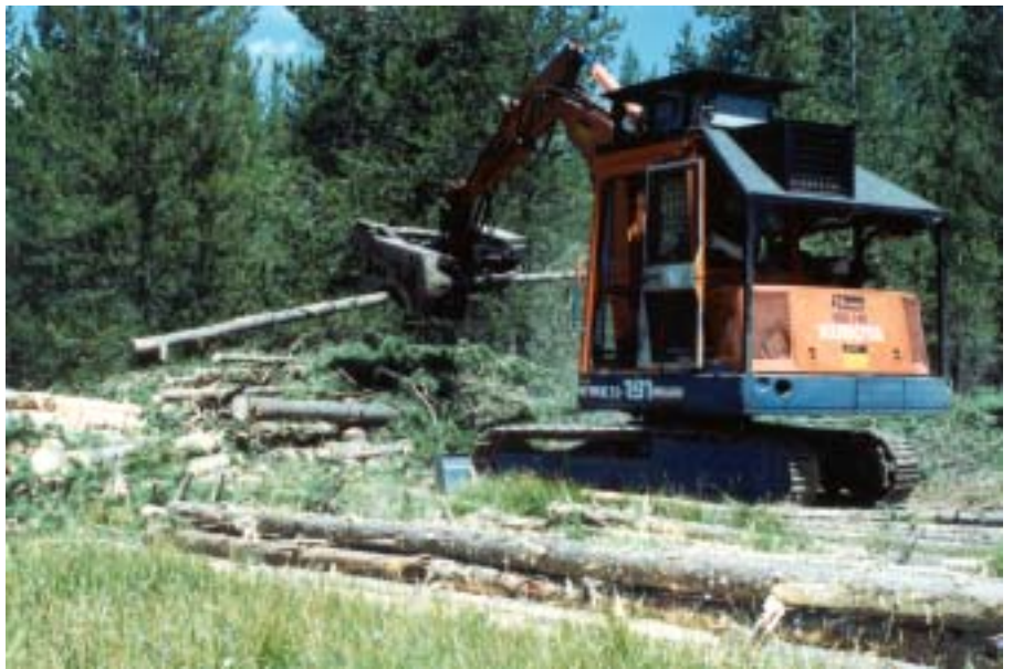
Figure 8—Processing at the landing with the Hahn HSG-140 head mounted on a Kubota KH-191 excavator.
