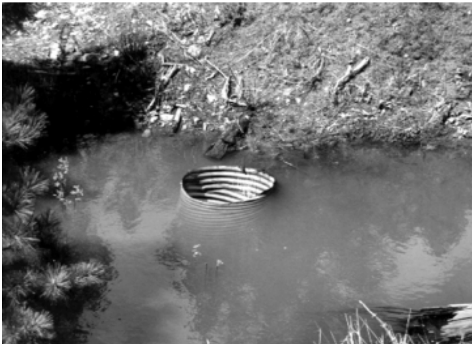
Figure 1—Elbow installed on cross drain to pond water and preserve sediment.
