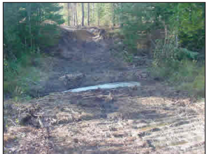
Figures 1 and 2—The temporary crossing in place and after its removal.
