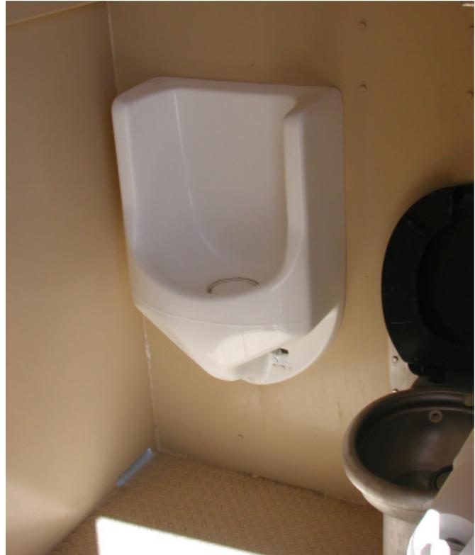
Figure 3—Waterless urinal and stainless-steel Microphor micro-flush toilet.
