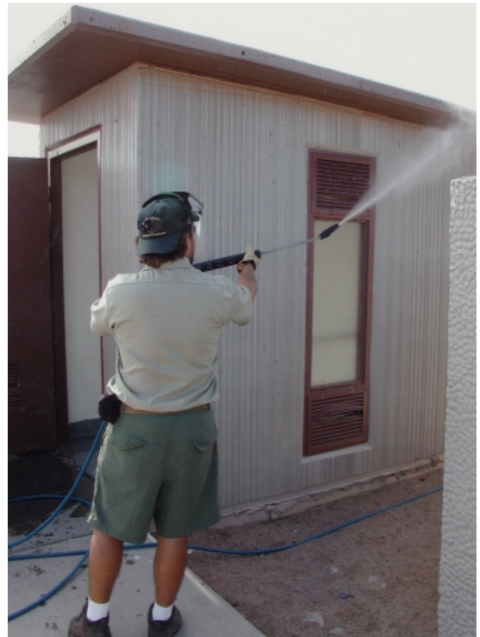
Figure 2—Cleaning the building exterior with a pressure washer.
