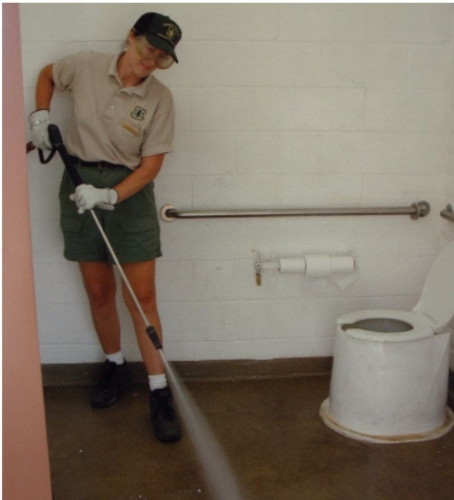
Figure 1—Cleaning the toilet interior with a pressure washer.
