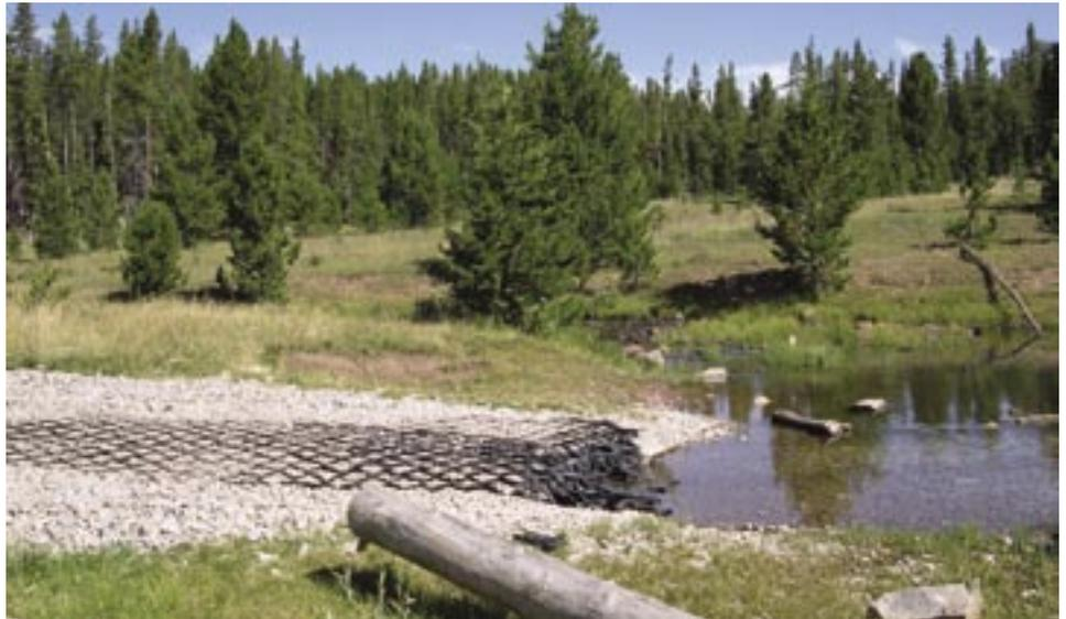
Figure A41. Looking upstream at erosion of one side of the ford in August 2004, 3 years after construction. Probably tire action and high flows have combined to pluck material out of the cells or undermine them. The ford is still intact and the geocells are covered by native bed material in the active channel.
