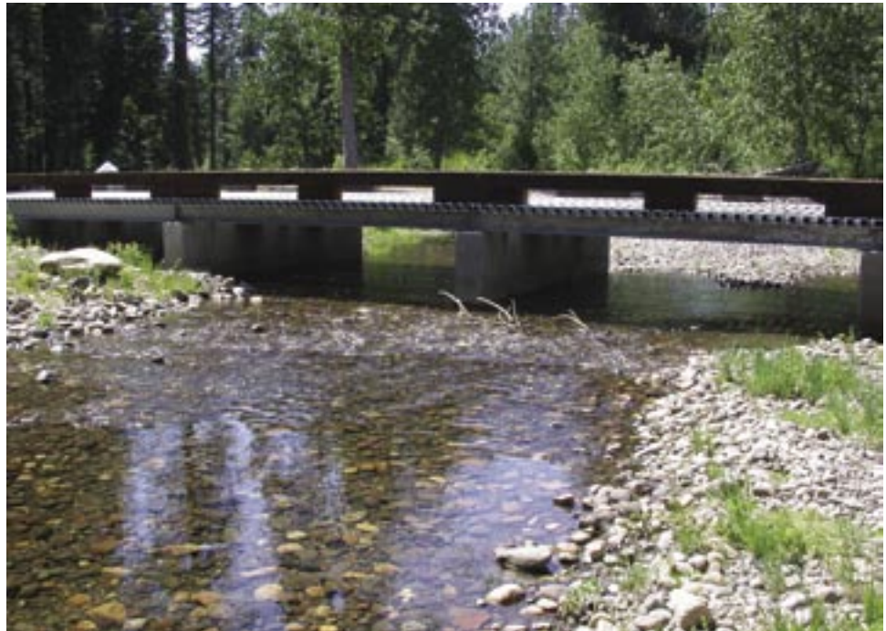
Figure A132. Looking downstream at the Capps low-water bridge. July 2002.
