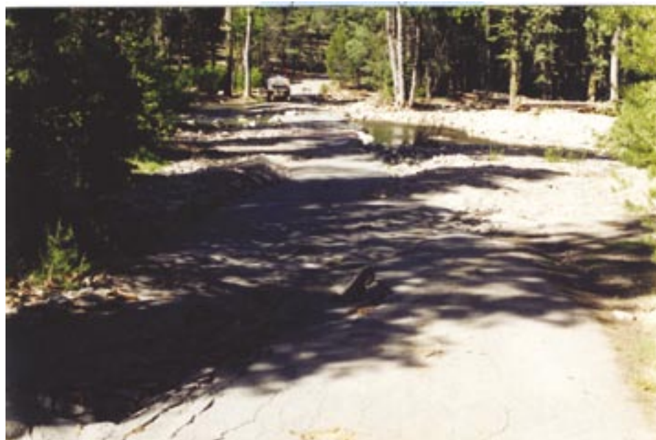
Figure A133. Capps ford after the 1997 flood. Flood flows spread out across the entire valley and road is washed out on far side.
