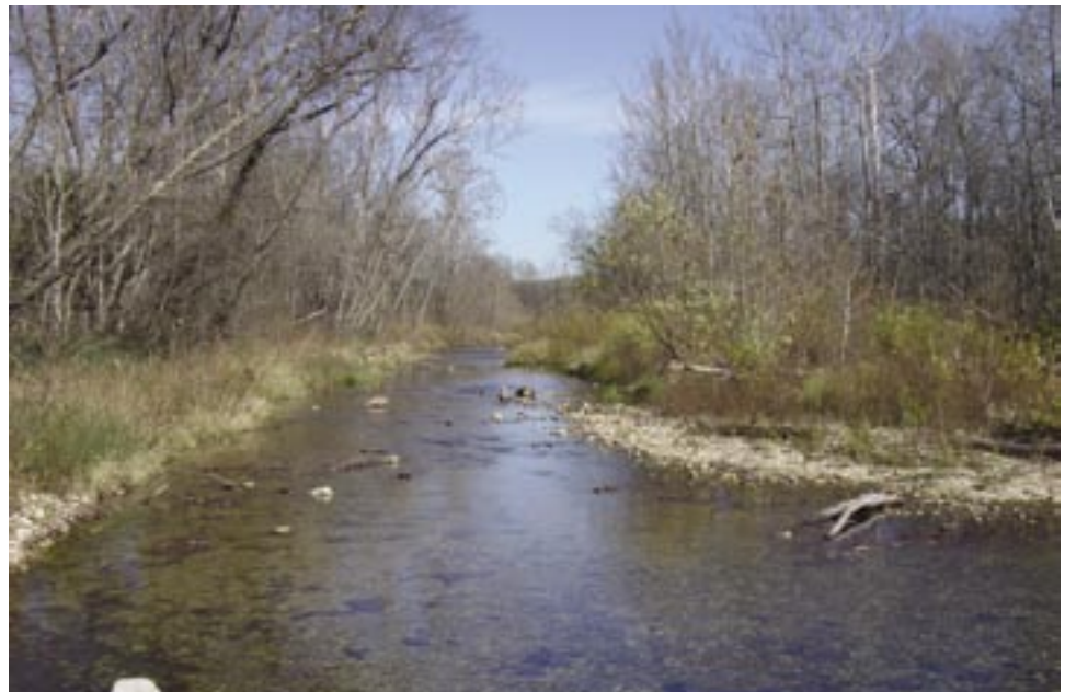
Figure A123. Looking downstream on Mill Creek from the box culvert ford.
