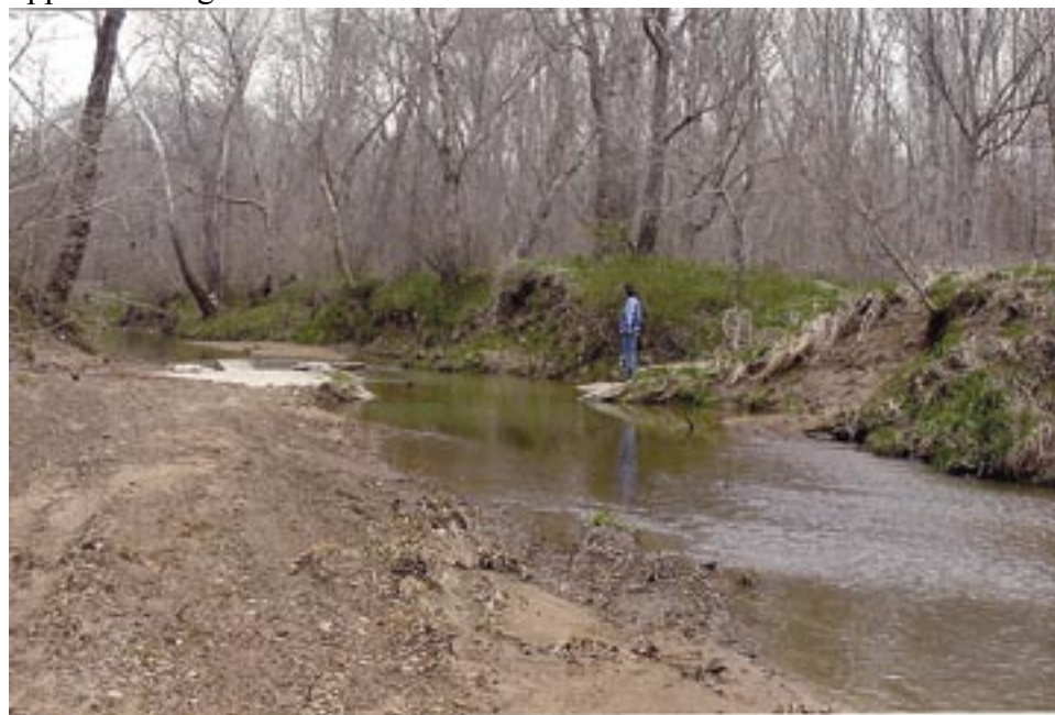
Figure A125. Looking upstream at failed Kinkaid Creek crossing, 2000. Stream slope is 0.3 percent.
