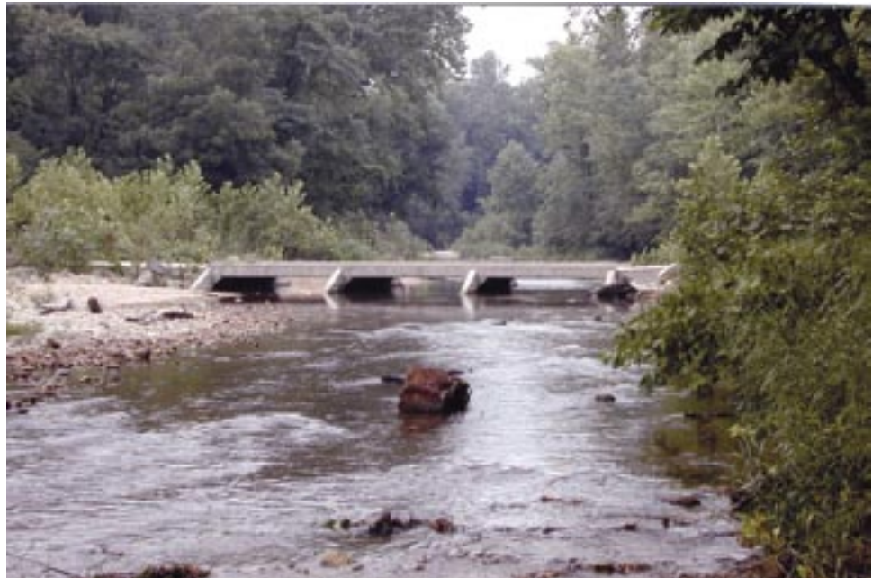
Figure A121. Looking upstream at Mill Creek box culvert vented ford, 2002.
