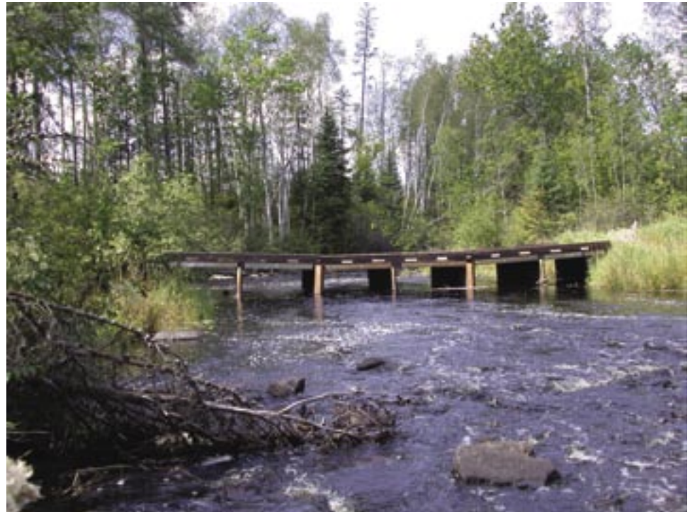
Figure A112. Stony River box culvert ford.
