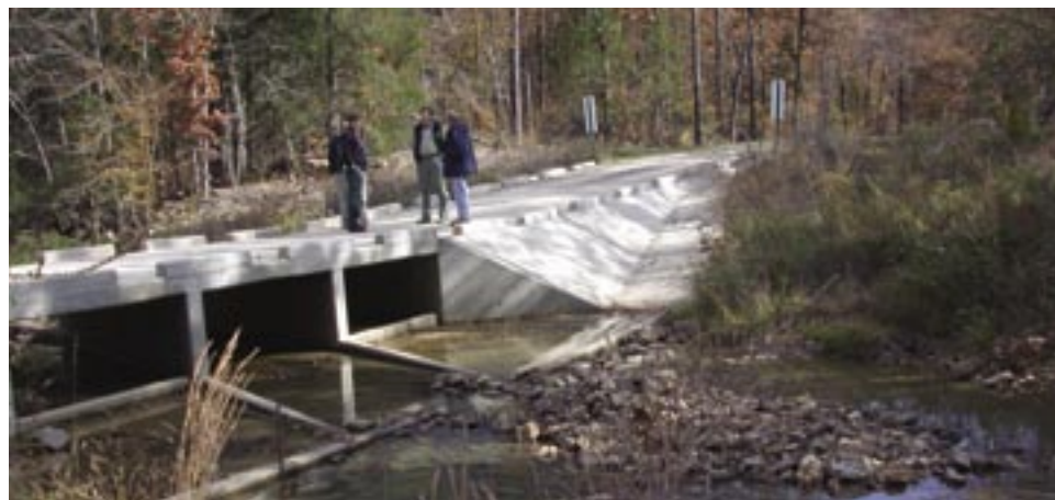
Figure A90. Looking upstream at the splash apron and backwater curbs.
