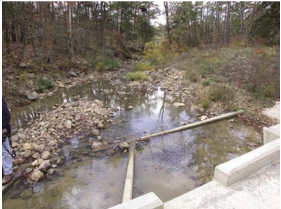
Figure A91. Looking downstream from ford. Note local channel widening.
