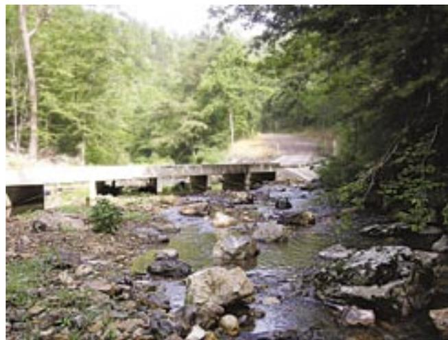
Figure 5.14—Long Creek embedded concrete box high-VAR ford constructed in 2005, Ouachita National Forest, Arkansas.
