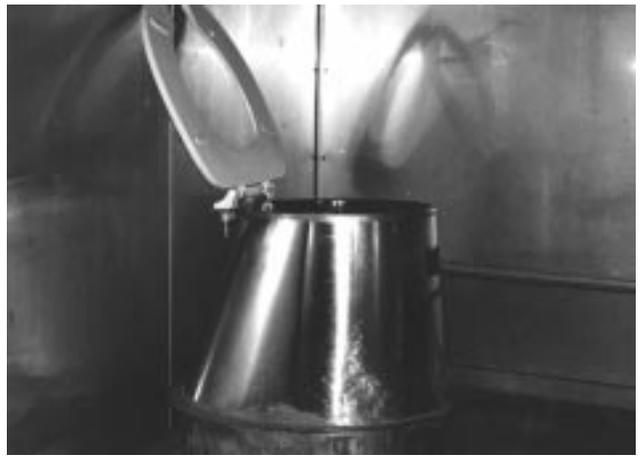
Figure 3—Concrete and riser cleaned with a full strength solution of Sub-Zero cleaner.
