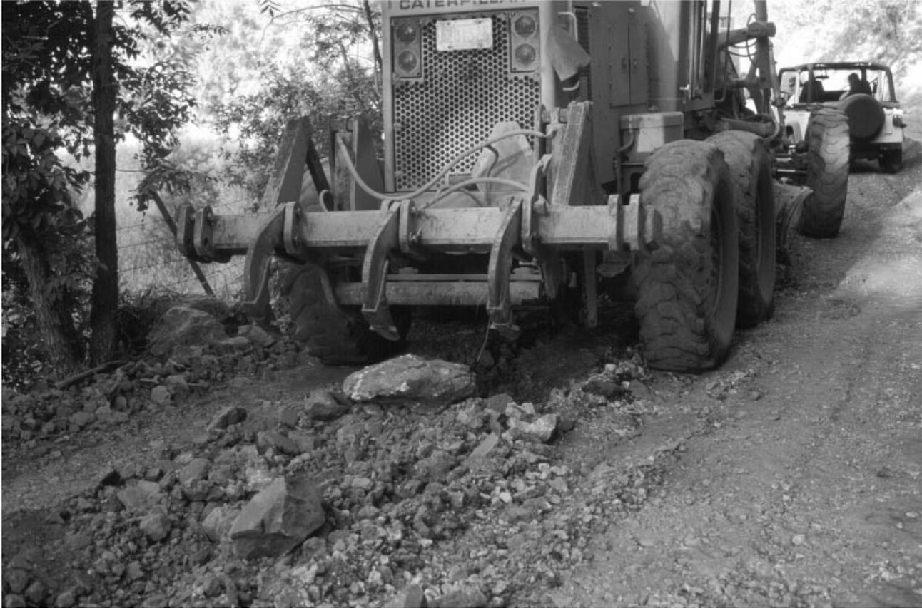
Figure 4. Grader ripping the road surface.
