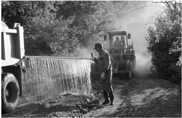
Figure 5. Watering windrow prior to crushing.
