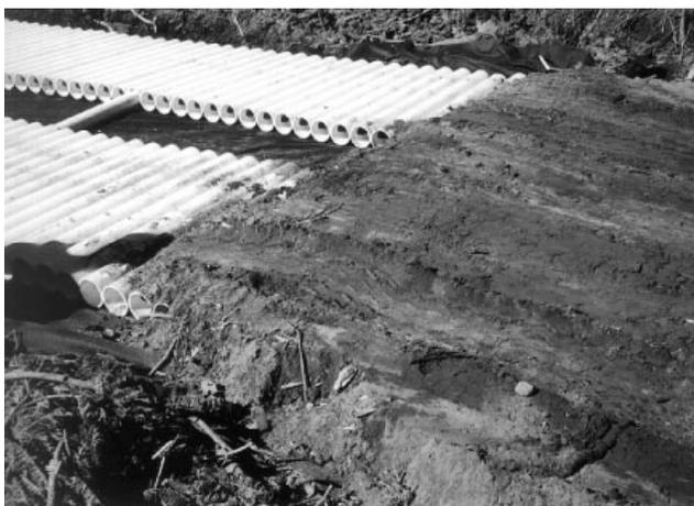
Figure 5. "Borrowed" soil ramps to the Plastic Road.
