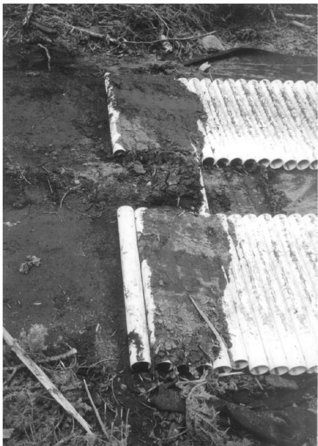
Figure 6. Plastic Road worked out of the soil ramp.
