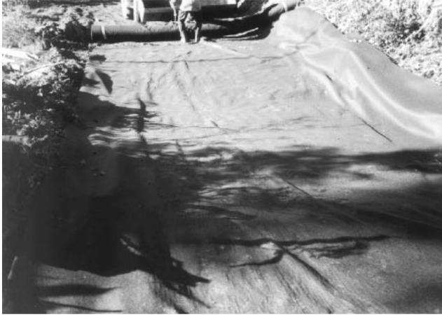
Figure 3. Geotextile underlayment to the Plastic Road.
