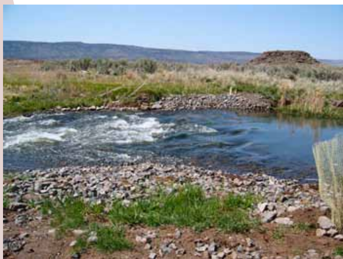
Figure 1. Rock riffle diversion control structure on the Malheur Wildlife Refuge, designed and photographed by author Dan Axness.
