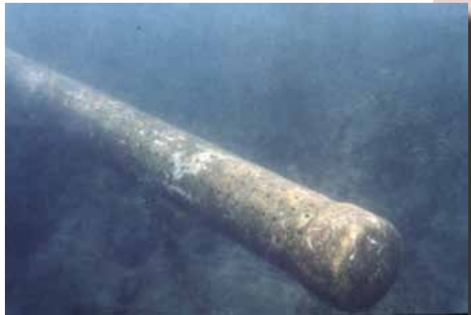
Perforated PVC screening water entering a pump. Photo by Kozmo Ken Bates, 2000.
