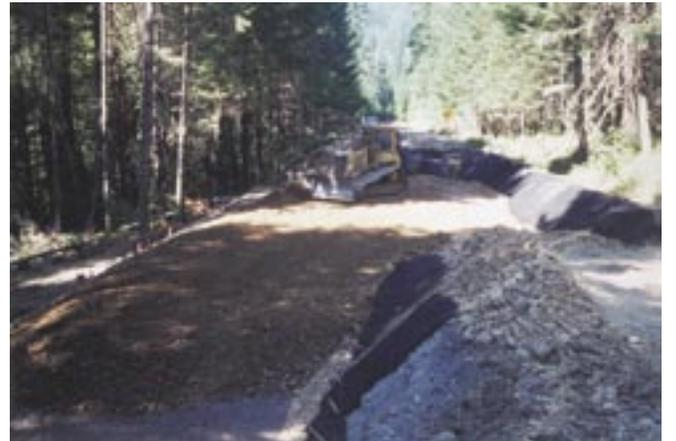
Figure 19—Backfill being placed over geogrid.
