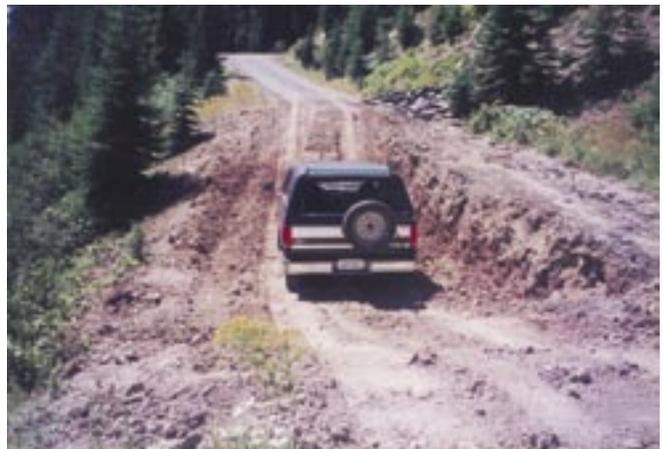
Figure 16—Excavation of distressed area prior to deep patch construction.
