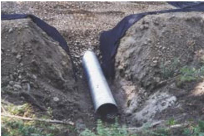
Figures 17a and 17b—Cutoff drain installation: 17a is parallel to road, and 17b is outlet pipe exiting fill.
