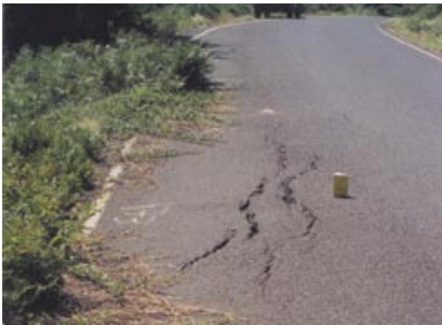
Figure 2—Pavement cracking as evidence of sidecast fill settlement.
