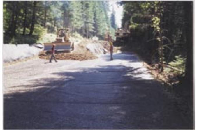
Figure 18—Geogrid layer placed prior to backfilling.
