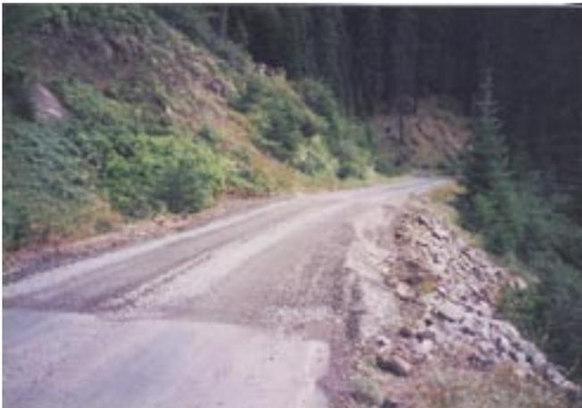
Figures 20a and 20b—Completed deep patches: 20a is paved, and 20b is left with gravel surfacing.
