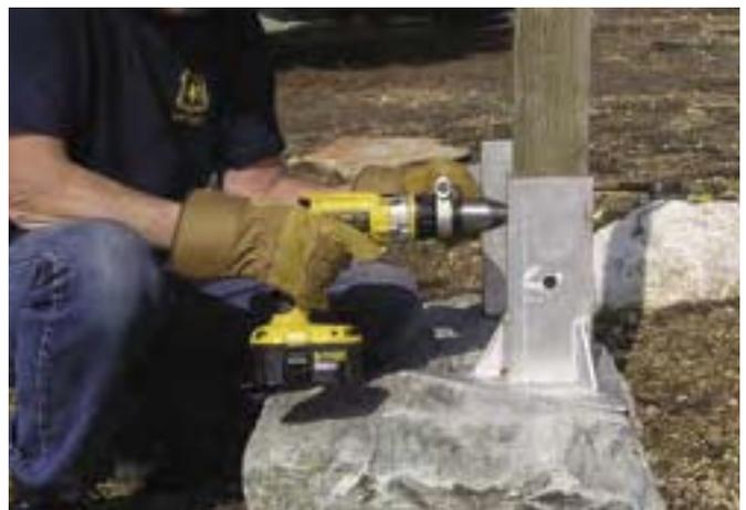
Figure 8—Metal-post base anchor.
