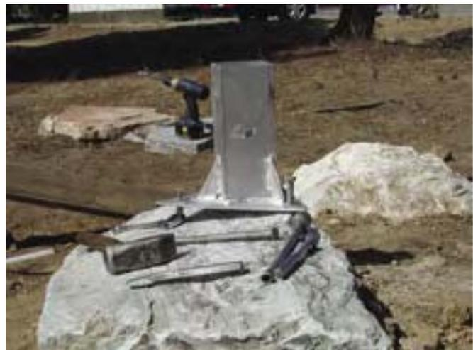
Figure 32—Metal-post base installation materials.
