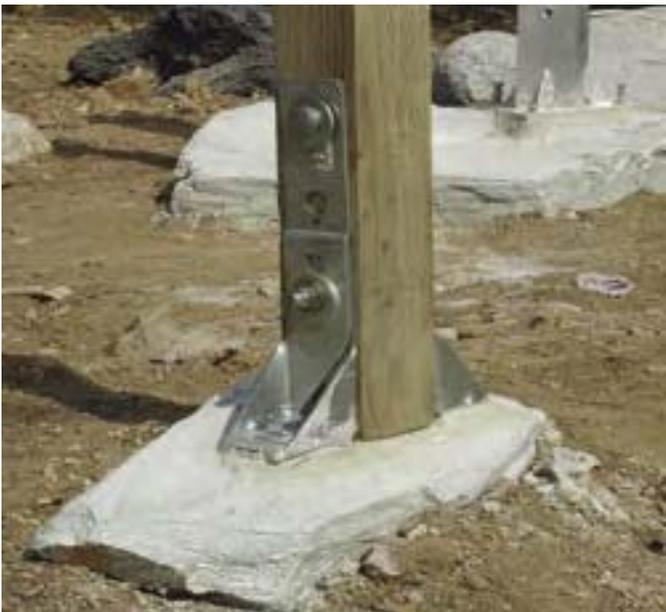
Figure 30—Holddown anchor installation.
