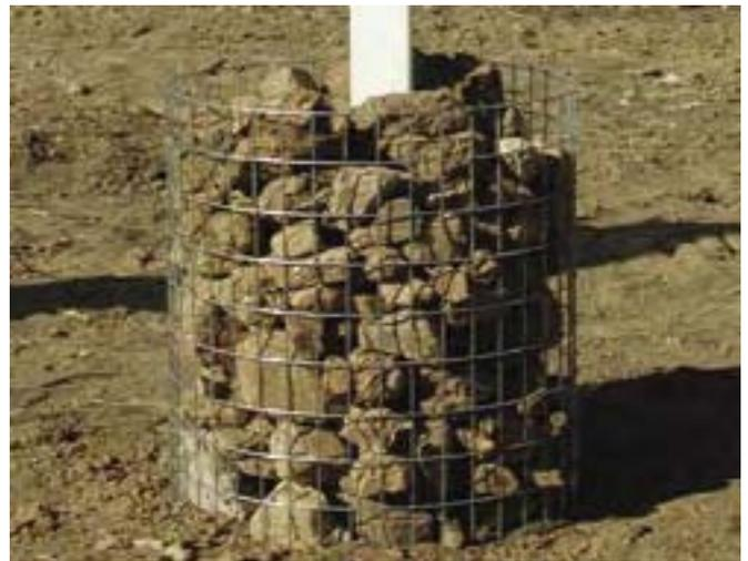
Figure 24—Completed rock basket for trail marker.
