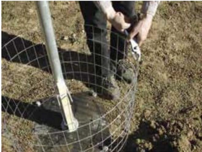
Figure 19—Fabricating the wire basket.
