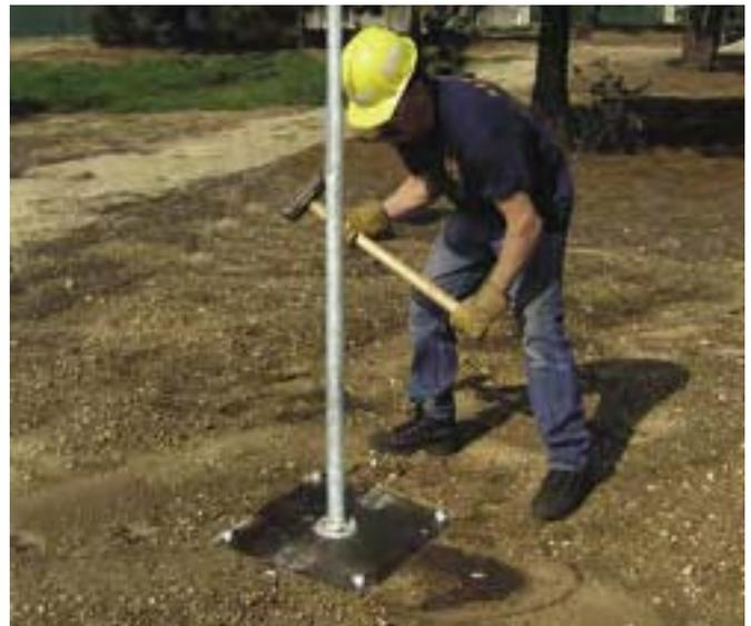
Figure 17—Staking the baseplate.
