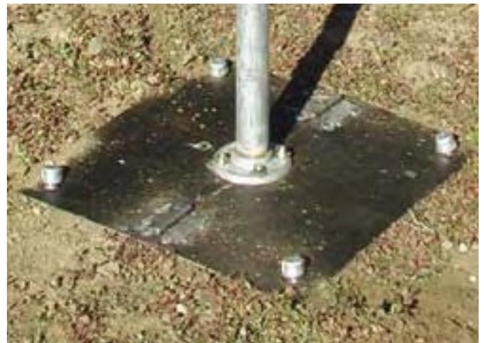
Figure 13—Split and hinged baseplate with pipe-flange connection.
