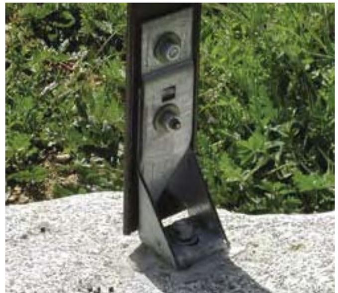
Figure 29—Completed anchor installation.
