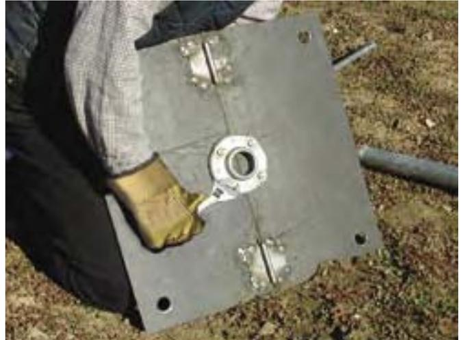
Figure 16—Attaching the pipe flange to the baseplate.
