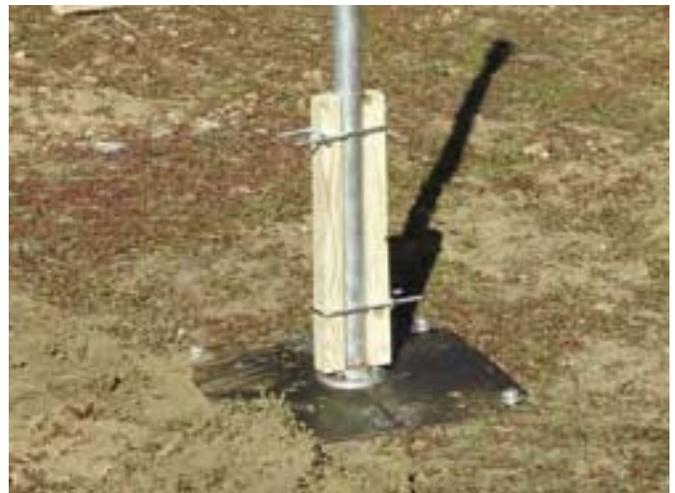
Figure 18—Using wood blocks to secure the pipe.
