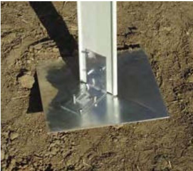
Figure 22—Attaching the trail marker to the base with angle brackets.
