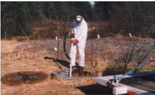
Figure 1—Vacuum pumping a vault.
