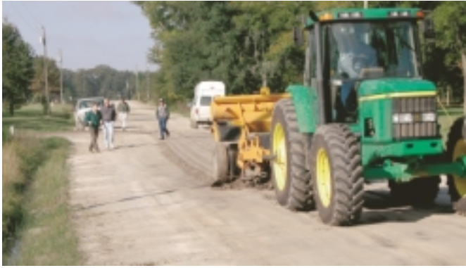
Figure 12—Grader pulled by a tractor.
