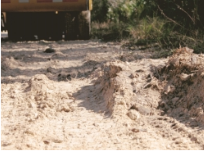
Figure 7—Elevation showing boulder top in road.
