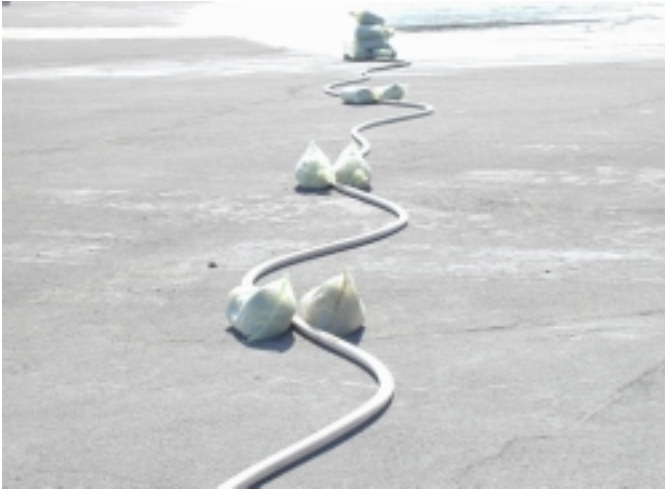
Figure 2—Sandbags are used to counter the reactive force during service testing.
