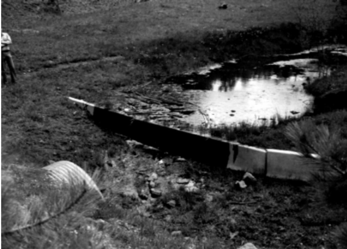
Figure 3—Jersey barrier gully plug.
