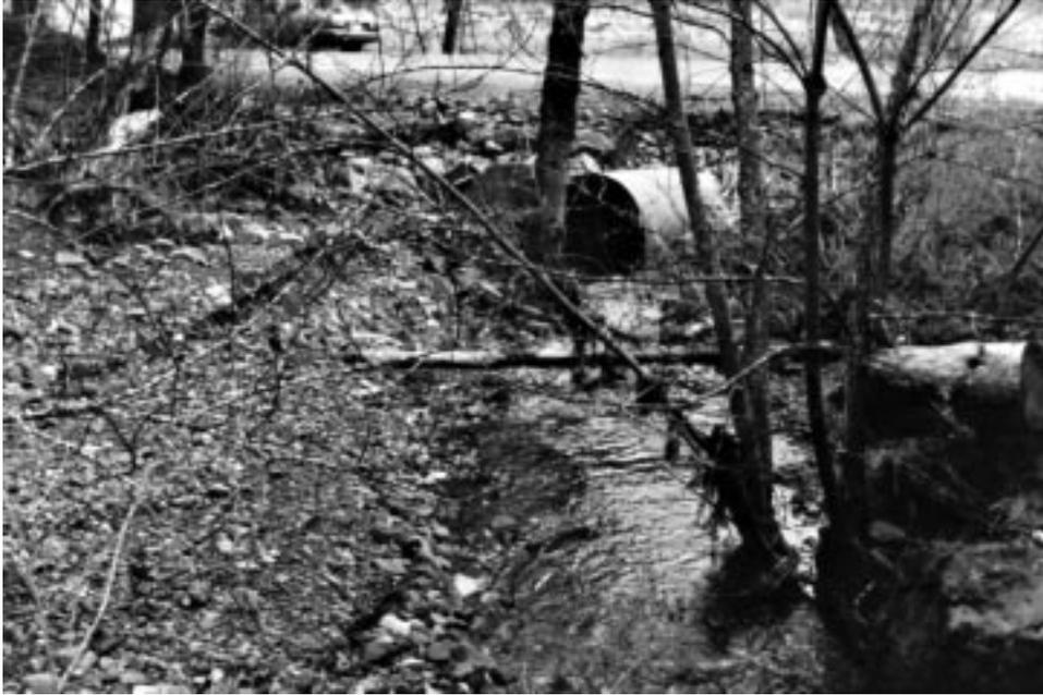
Figure 1—When compared with the bed width, the zone of average annual bedload transport, this culvert is undersized. Hydraulic calculations show this pipe unable to pass a 10-year design discharge. Also note terrace development. Such physical features often coexist and provide evidence for inadequately sized culverts.
