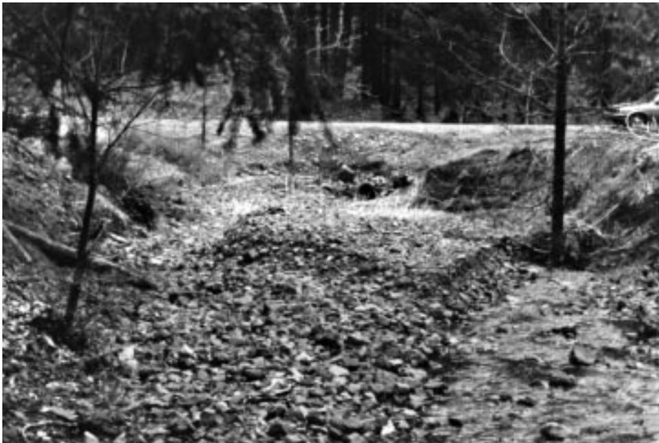
Figure 3—Terraces upstream of the culvert inlet indicate past ponded conditions. Channel dimensions and hydraulic capacity of this culvert should be checked.
