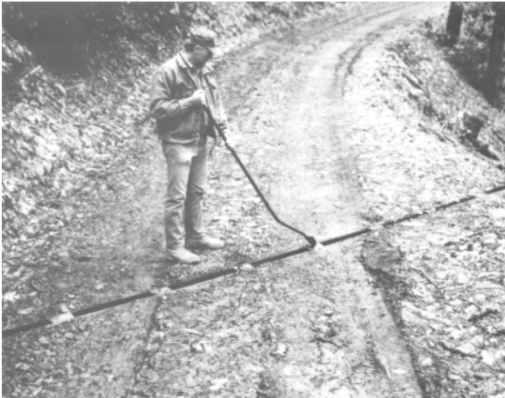
Figure 3—A tool for cleaning open-top pipe culverts is made by bending a 5-foot (1.5 m) piece of 3/4-inch (19 mm) pipe two ways and welding to it a 4- by 5-inch (100 by 127 mm) shaped piece of metal cut from a pipe.
