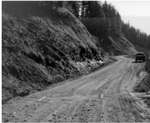
Figure 4a and 4b—Two views of the Portable Road Spillway.
