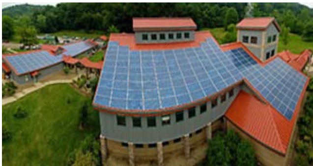
Solar Expansion Project at the Wayne National Forest Headquarters building (Photo by Alex Snyder)
