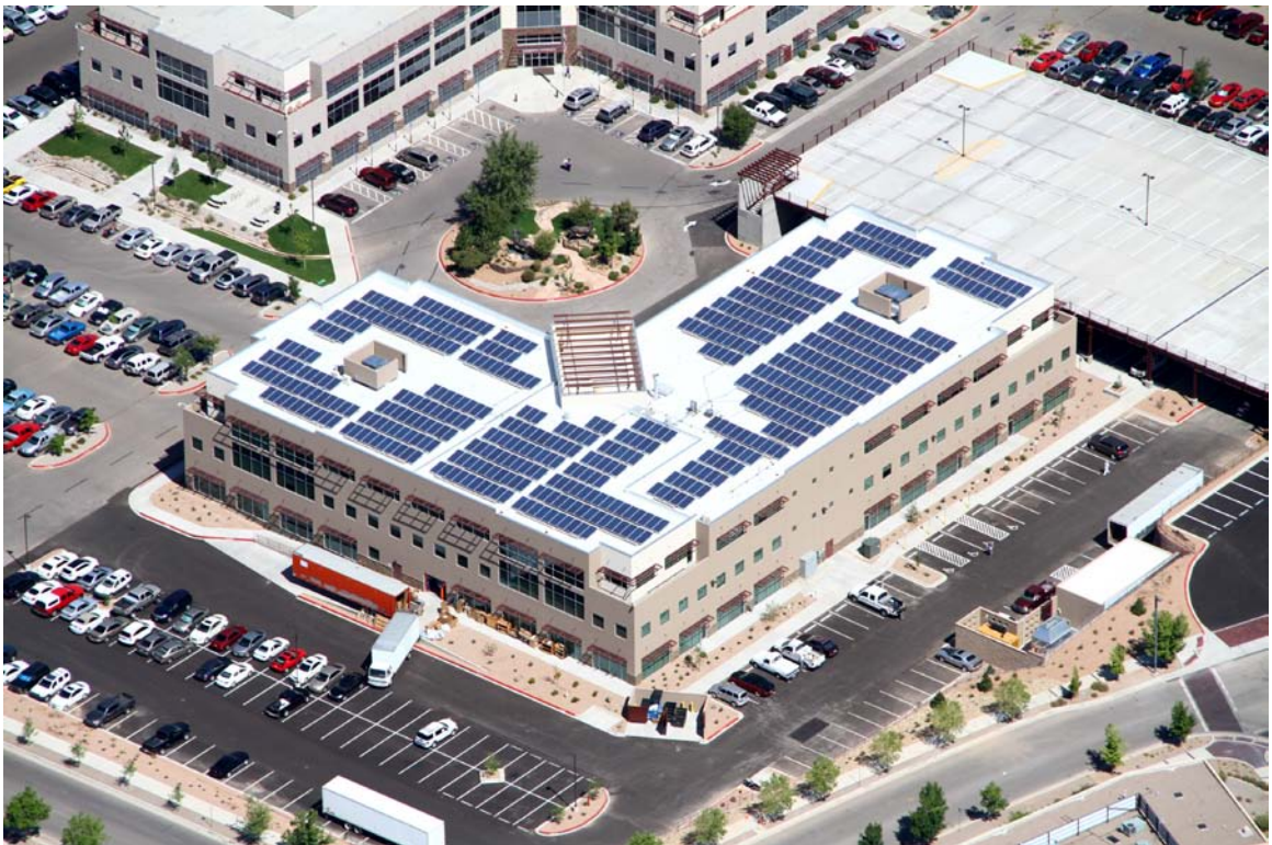
Aerial view_ photovoltaic array
