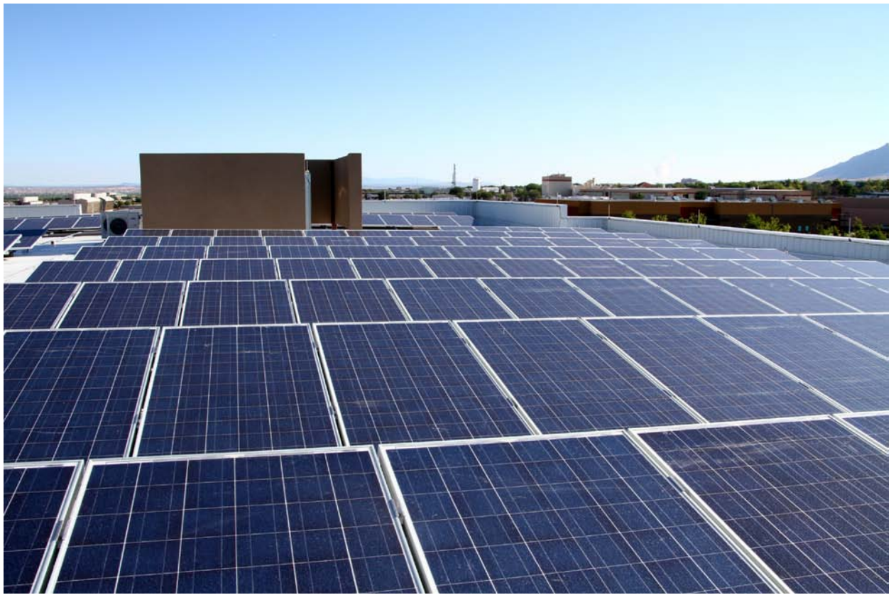
Roof view_ Photovoltaic array
