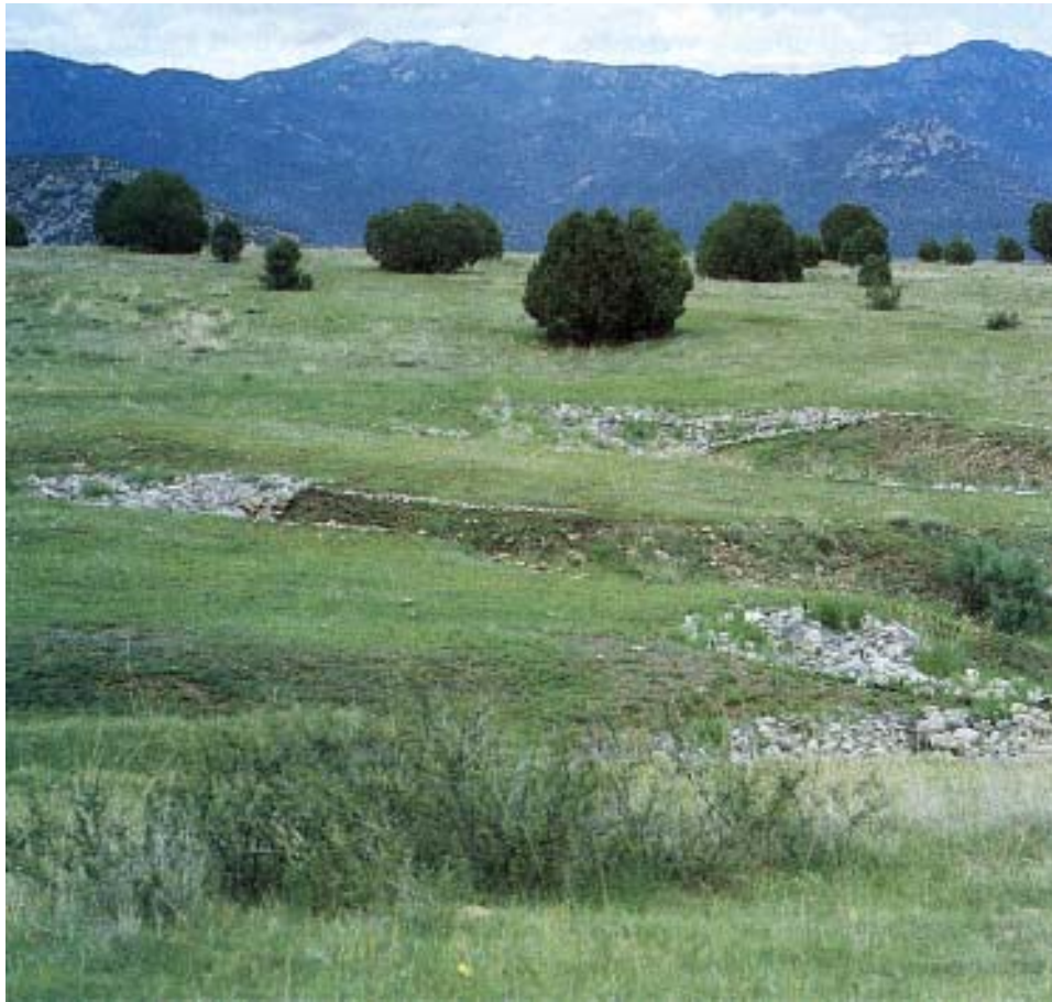
Figure 2. Protecting unstable stream channels by placing rocks on channels walls.
