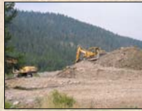
Floodplain restoration work on dredge tailings in progress
