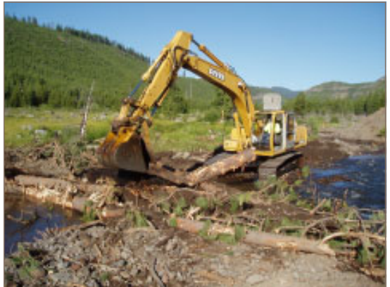
More than 2,100 trees were used to create log jams and pool habitat which in turn improved wildlife and fish habitat
