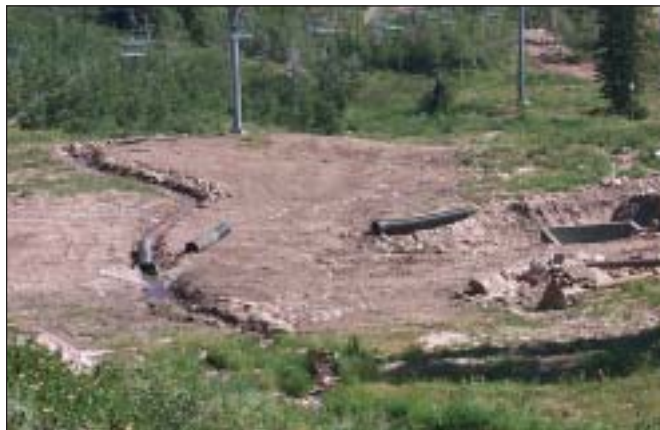
This stream has been moved away from new impacts and into the original channel that existed before the chairlift and ski run were constructed.
