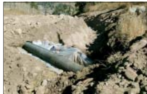
Several culvert sections can be joined where longer temporary stream crossings are required. Be sure to use plastic sheet lining to keep water leaks out of the trench.
