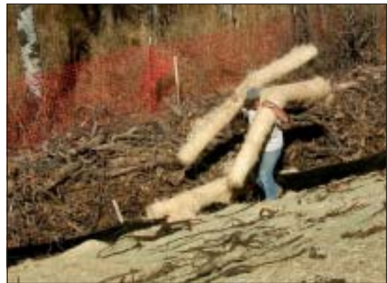
Blankets can be combined with silt fencing to provide added protection next to streams and wetlands.
