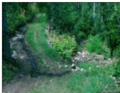
Road cut slopes can intercept and expose subsurface water.
