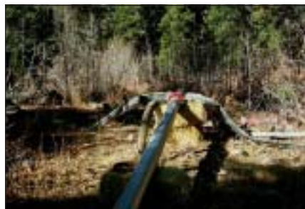
Innovative manifolds and hose lays are effective methods for dispersing high volumes of water from well production tests.
