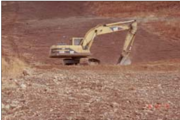
Waterbar installation by trackhoe excavator.
