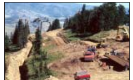
To reduce corridor width and disturbance, long sections of pipe can be connected at a central staging area and lined downhill.
