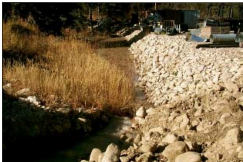
Sediment pond outlet ditches should be armored with rock to prevent scouring. Step pools in the outlet ditches allow even more sediment to settle out.
