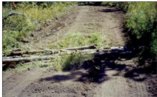
Logs can be used instead of culverts and fill to provide a temporary stream crossing for heavy equipment access across intermittent and ephemeral channels.
