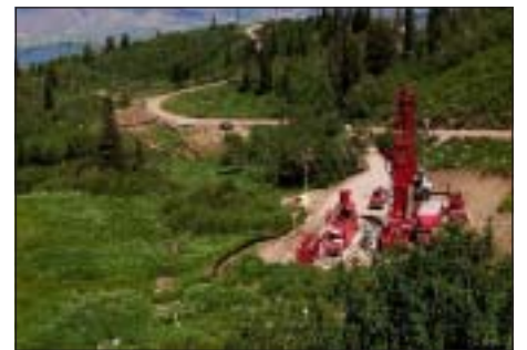
Water source wells are often developed in close proximity to wetlands and springs.
