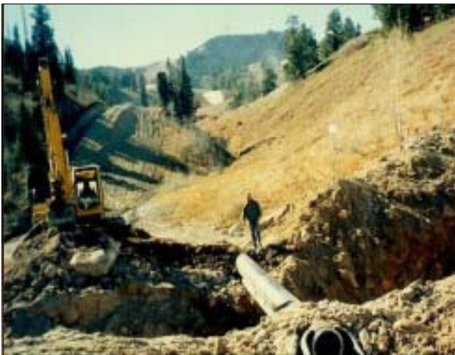
Wherever a trench cuts through a channel, a temporary crossing must be installed to keep the stream out of the trench.
