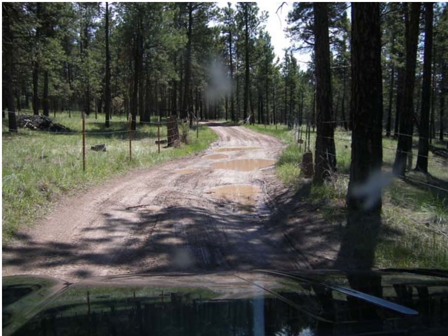
Figure 4. View of existing road in timbered area.
