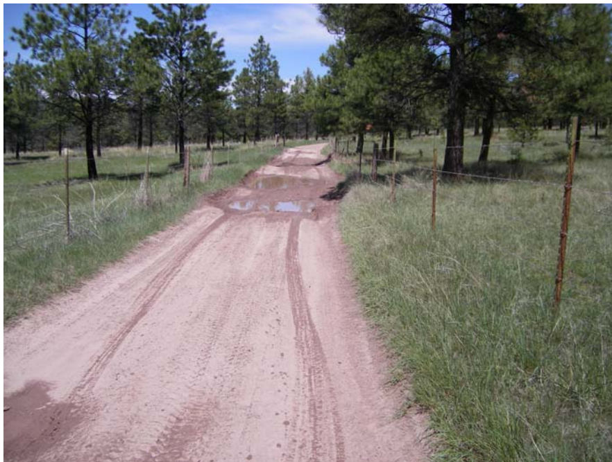
Figure 2. Typical mudhole on existing road. Note the closeness of the fences on each side of the road.
