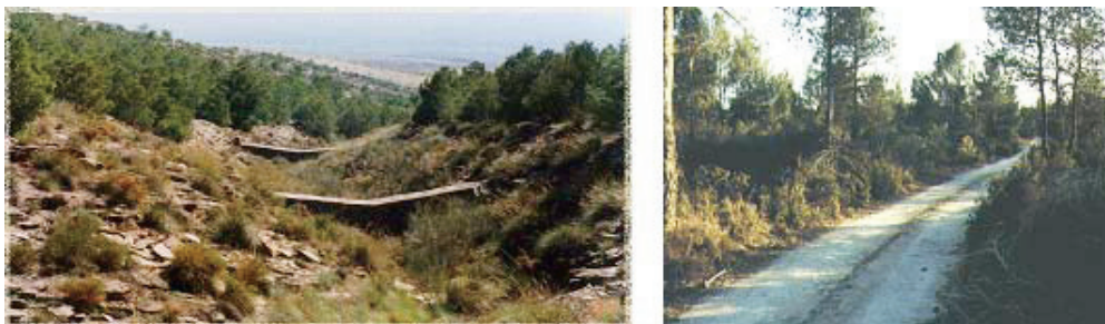
Figure 3 —Hydrological works and road improvement in the area of study.
